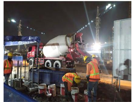
*Preparation of Admix slurry to be added to concrete truck*
