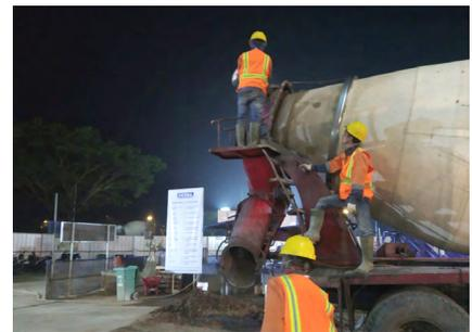
*Mixing Xypex Admix into the concrete truck*
