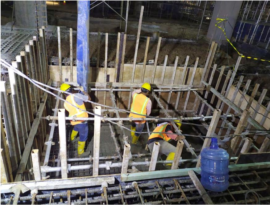
*Pouring Concrete with Xypex Admix for the 'Grey Water' tank*
